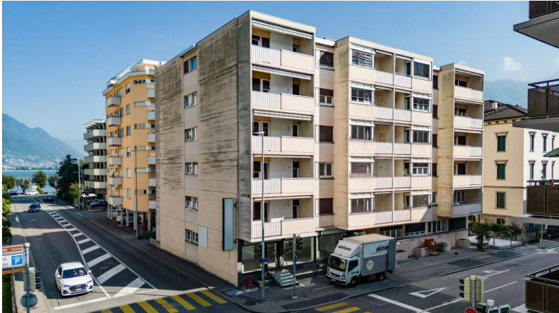
Photo before refurbishment
